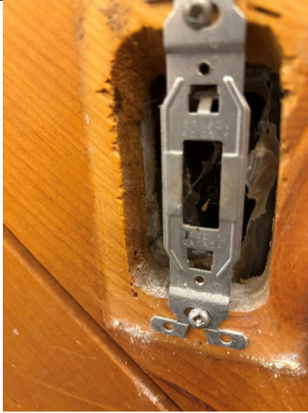
Photo 4: View of wood panelling over top of gypsum board in community hall.
